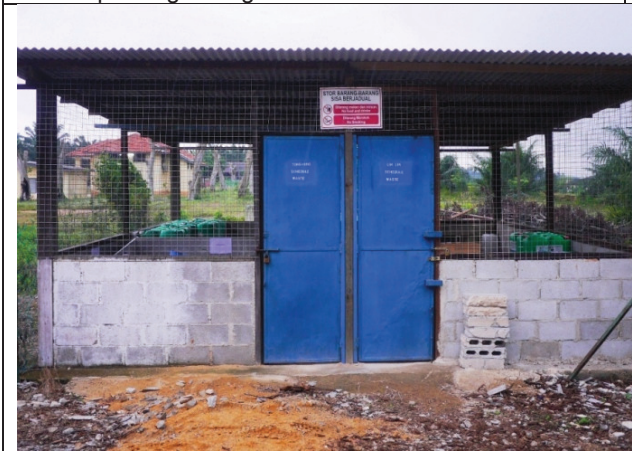
Sin Lian estate: Schedule waste store
